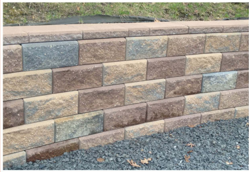
ALLEN BLOCK RETAINING WALLS
